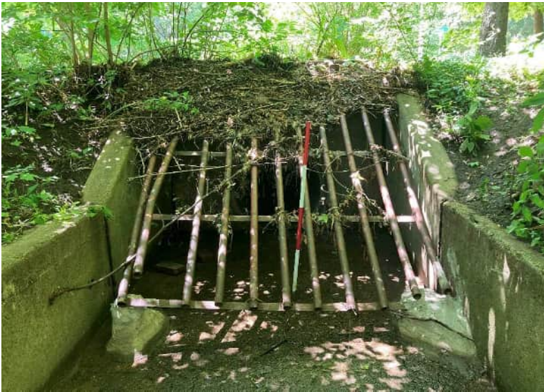
Photo 7 Channel outlet 42" RCP heawall, socket end 7' x 30" Rectangular channel
