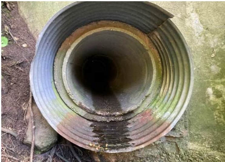
Photo 14c Right outfall- 24" RCP Concrete pipe with CMP sleeve extension
