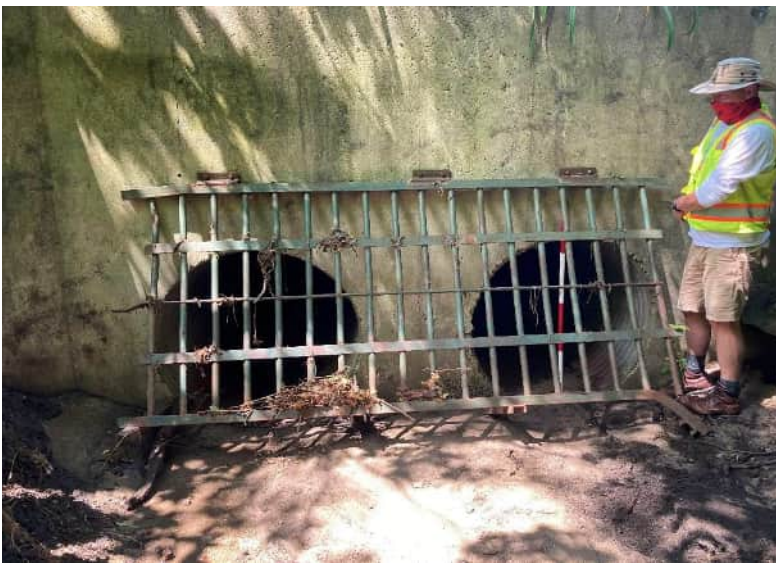
Photo 11 Dual 42" CMPs Square Headwall
