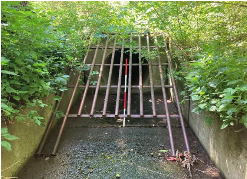
Photo 10 Channel outfall 48" RCP
