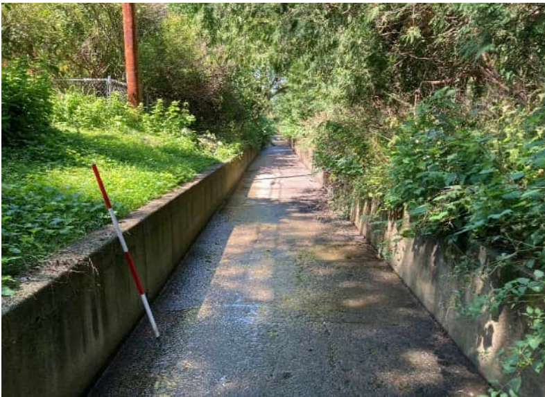
Photo 17 7' w x 30" h rectangular channel Clean and very good condition
