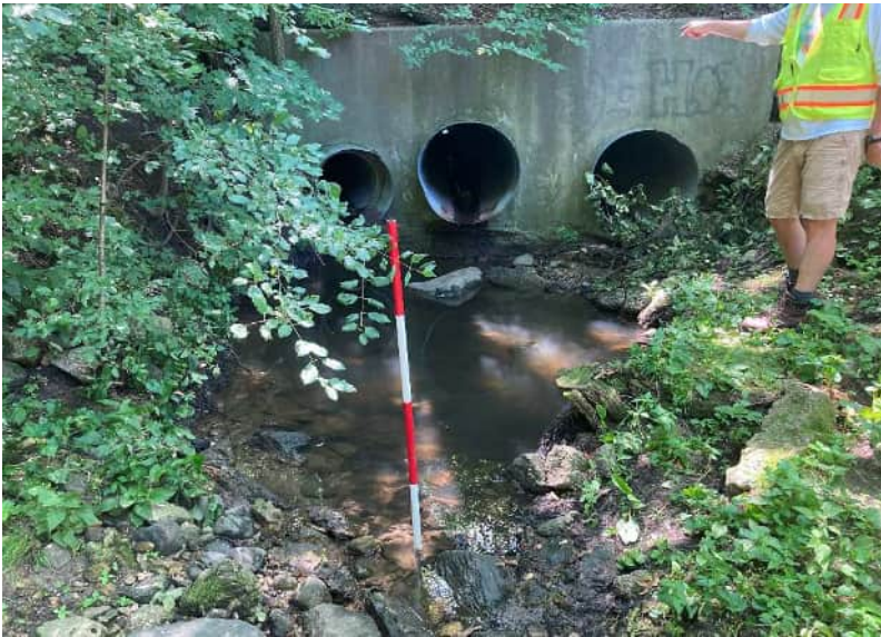
Photo 14 Outfalls into channel Left - 36" CMP Middle - 36" CMP Right - 24" RCP (end sleeved CMP)
