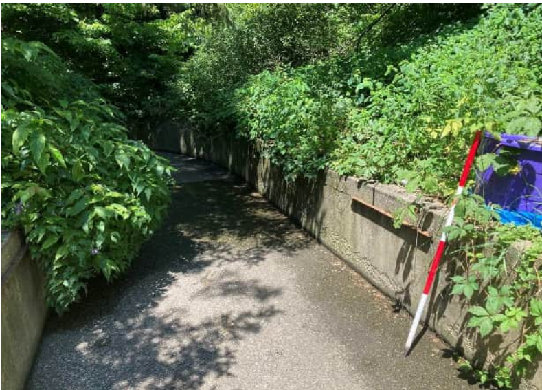
Photo 8 First bend in channel upstream of outlet Note cantilever for bridge abutment
