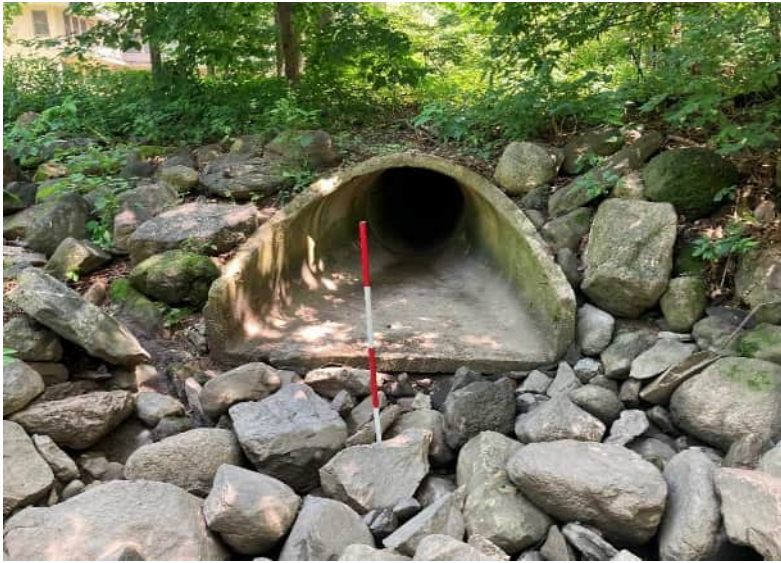
Photo 5 Primary outfall 36" RCP FES
