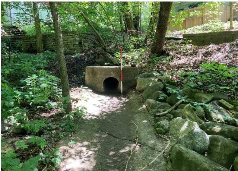
Photo 3 Outfall on left side of channel. 18" CMP
