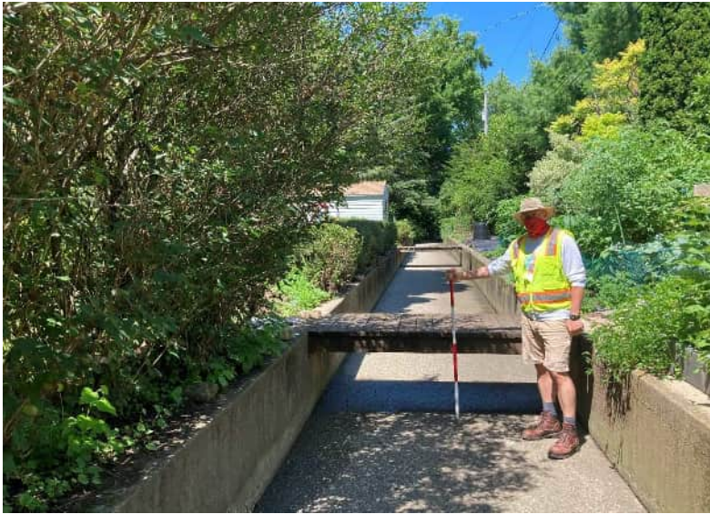
Photo 9 7'w x 20" h channel with two wooden bridges
