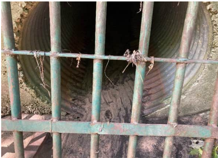
Photo 11b Sediment build-up on right channel outlet
