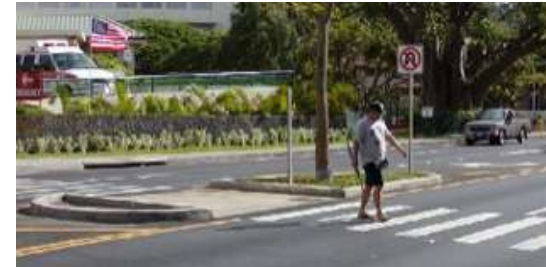
Pedestrian refuge island with crosswalk
