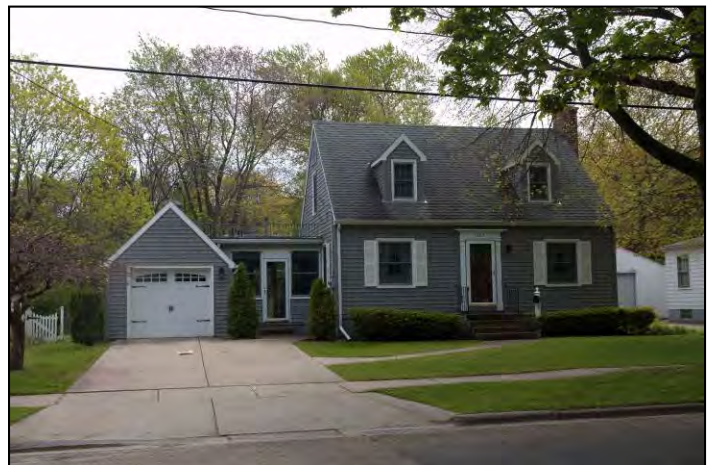
Example of cottage architecture.
