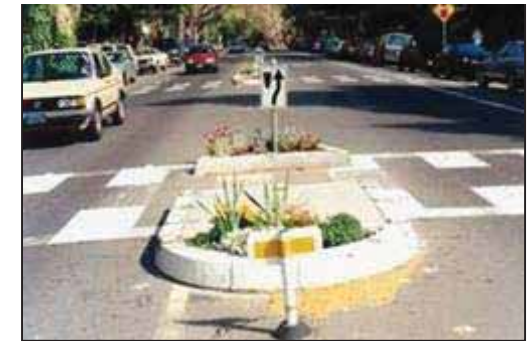
FIGURE 4.7 Pedestrian crossing should be clearly identified
