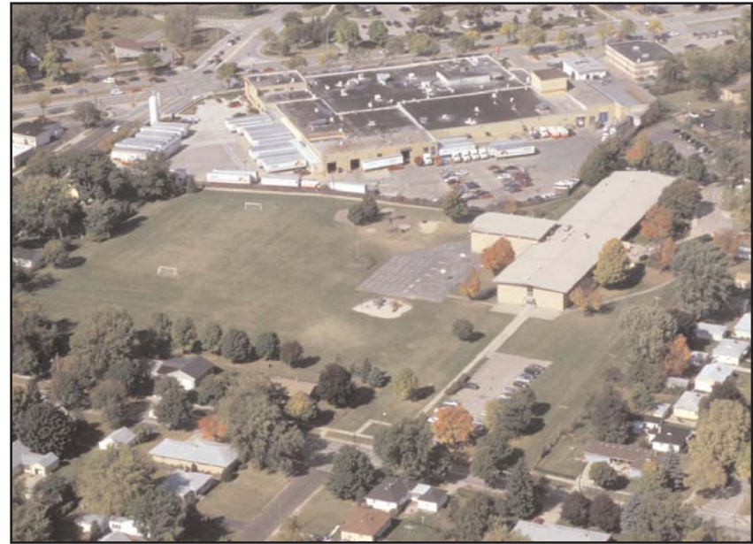
View of Hawthorne Elementary School looking north
