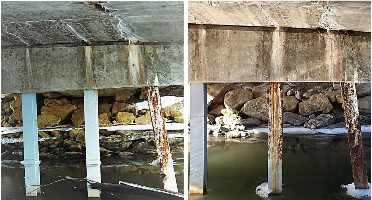
Corrosion of former Highway 19 Yahara River Bridge. March of 2013 on left, December of 2019 on right. Stalactites form at the largest fracture every winter and slowly dissolve over the remainder of the year.
